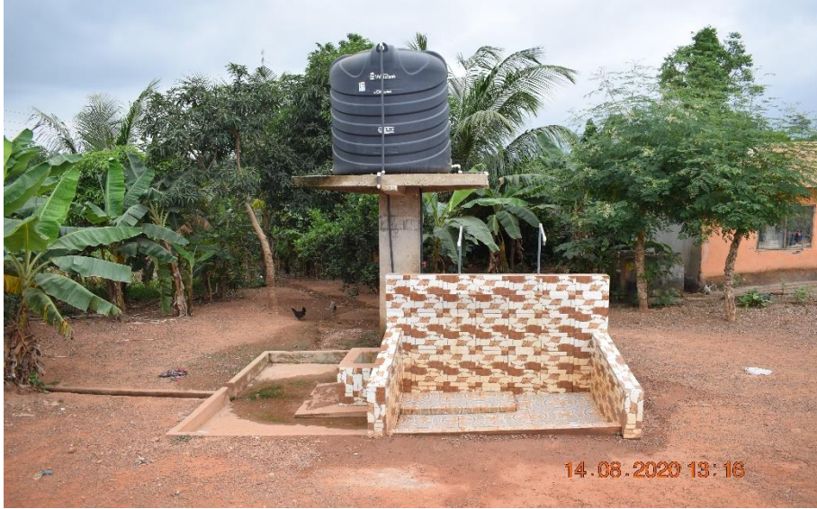
39. MECHANISATION OF 5 NO. BOREHOLES AT AFOAKO, NYAMEBEKYERE, ABOO, NTOMEM AND ADINKRA
